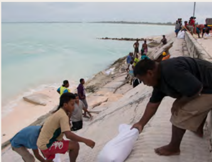
Sandbagging a hole in the Betio causeway, Kiribati eroded by waves from cyclone Pam.
