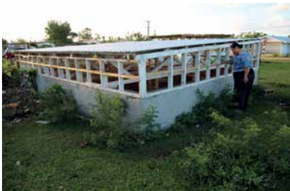
Restoring an emergency water storage tank in Ha’apai, Tonga.
