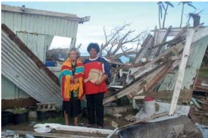
Mele'ana and 'Ana Kofe in the remains of their home in Lifuka after cyclone Ian hit Ha'apai in Tonga in January 2014.
